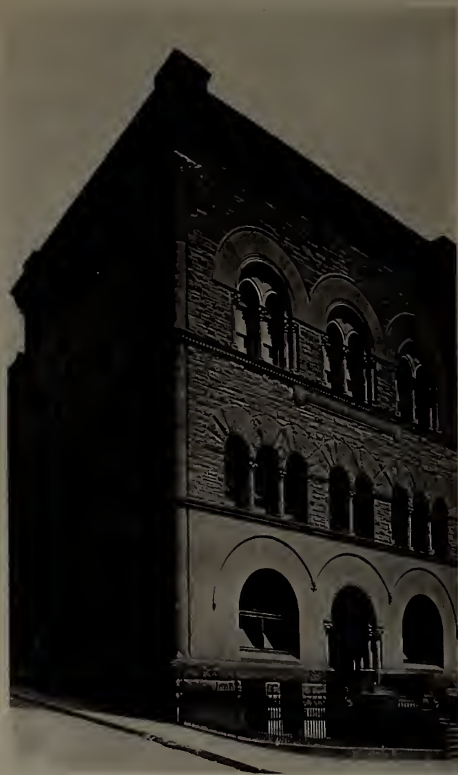
UNITARIAN HEADQUARTERS, Beacon Street.
